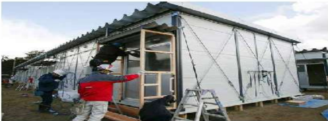
Figure 10. Demountable temporary housing (Kasetsu Jutaku) in Japan following the 2011 earthquake. Source cited in the underlying research: House of Japan (2011). The example illustrates the distinction between demountability and simple portability.
